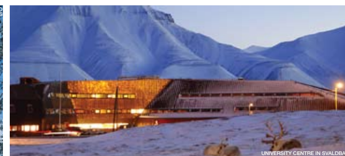
UNIVERSITY CENTRE IN SVALBARD PHOTO: NILS PETTER DALE, ARCHITECTS: JARMUND / VISSNES AS ARKITEKTER MNAL
